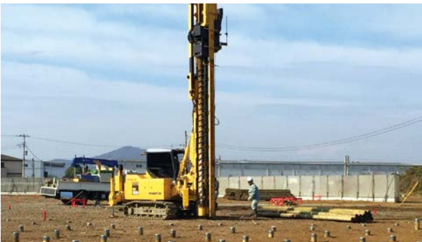
Ground improvement using lumber that has undergone preservation treatment
