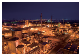
JCM Project: Chlorine production plant in Saudi Arabia equipped with high-efficiency electrolytic cells
