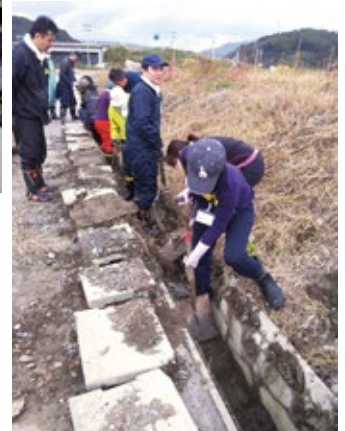
Removing dirt from gutters
