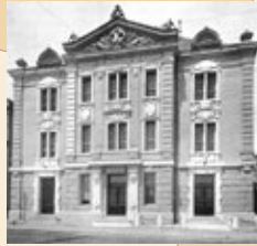
1911 Former Kobe Head office 'Nichigo-kan,' which was completed Still popularly used as a commercial building
